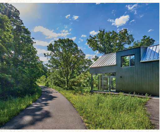
Photos: (Top to bottom) The Ryerson Education Center is situated in a woodland clearing north of the preserve's entrance road. • Construction crews worked within limited space to protect the surrounding trees. • The 0.2-mile paved Kevin and Jean Froeter Learning Trail is fully accessible.
