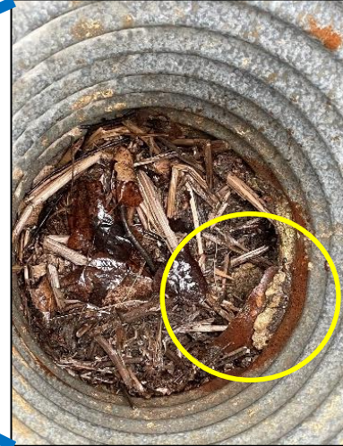
Photo 9 – Inside CMP control structure, SE pipe outlet observed
