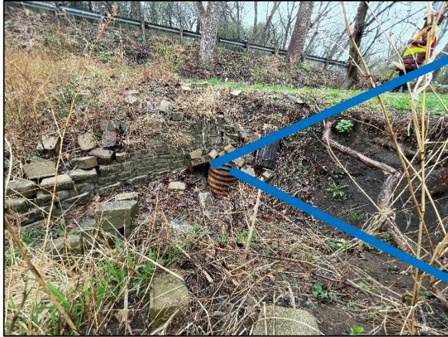
Photo 8 – Control Structure at NE corner of pond
