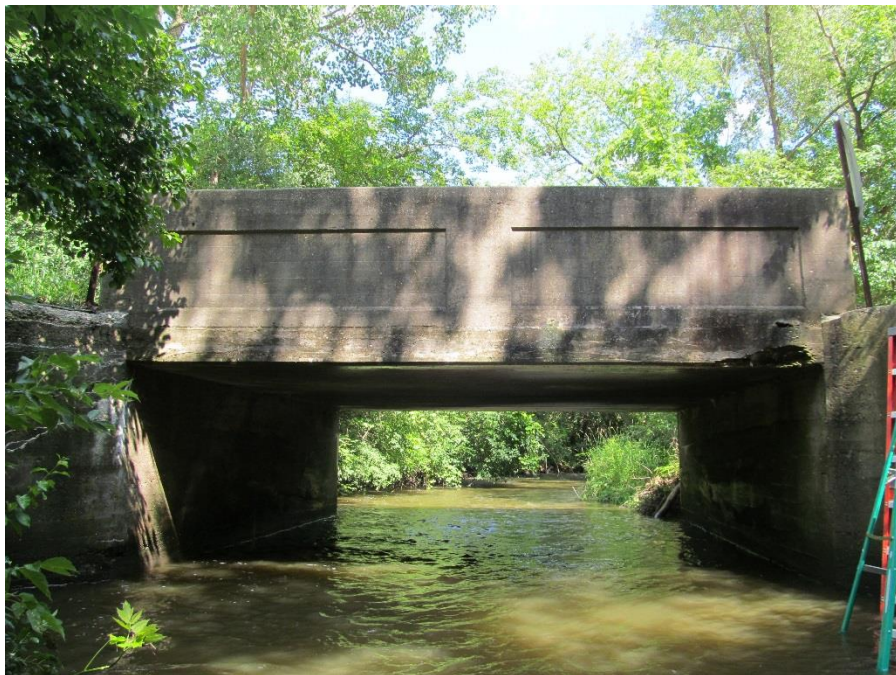
Figure 2. Bridge elevation looking east.
